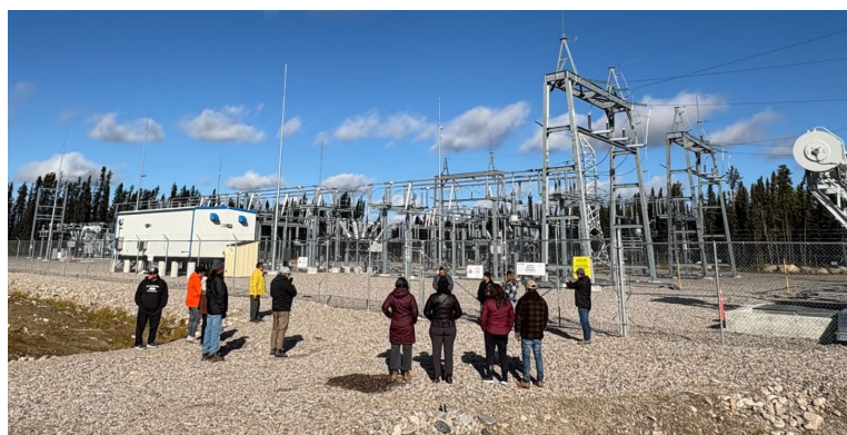
A substation blessing was also completed for Muskrat Dam Substation E on October 15, 2025.
