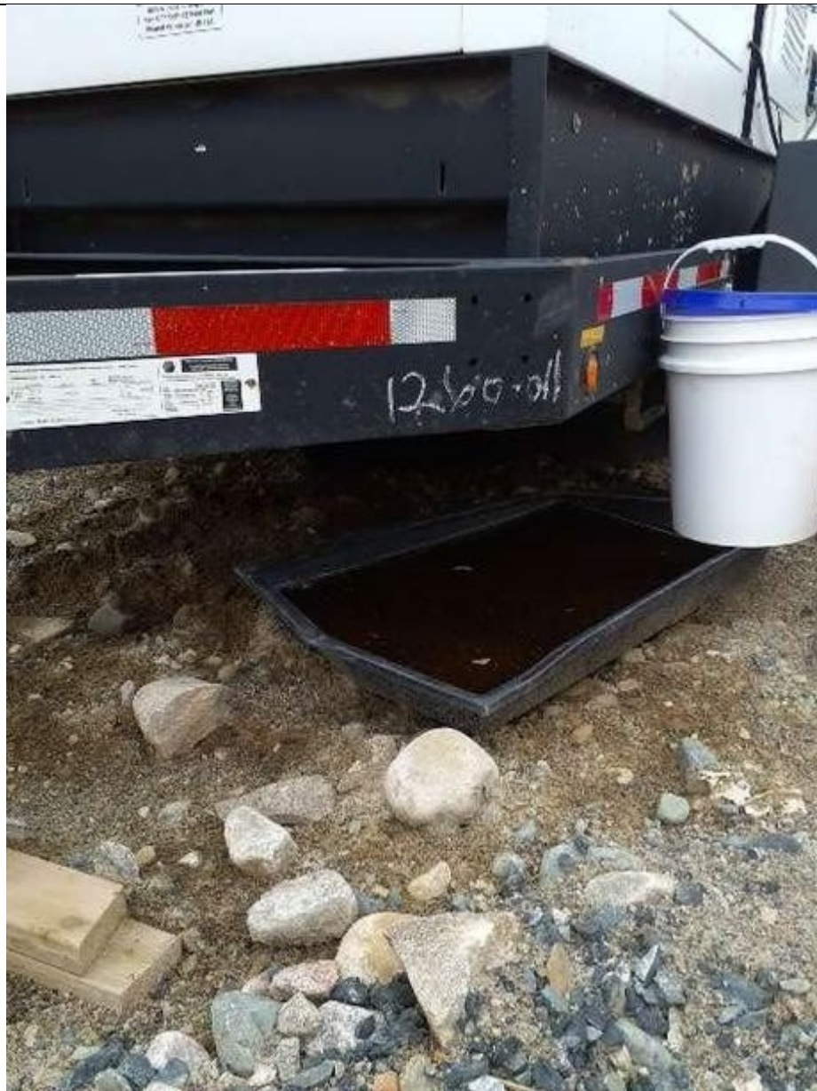
Fig 5 Caption: Filled spill trays under generator
