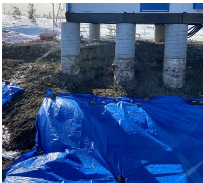
Substation P Excavation Site. Tarp used to help thaw frozen ground underneath.
