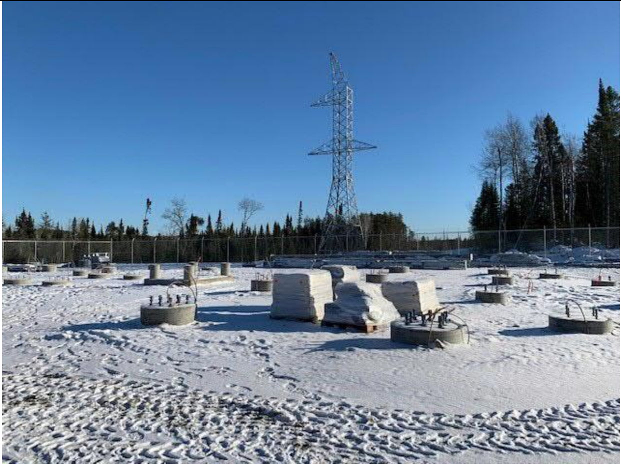
Substation A Progress.
