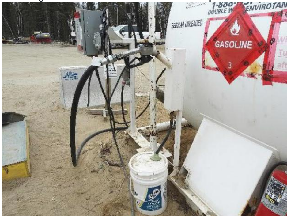
Figure 4: Gas nozzle holster with containment container in place
