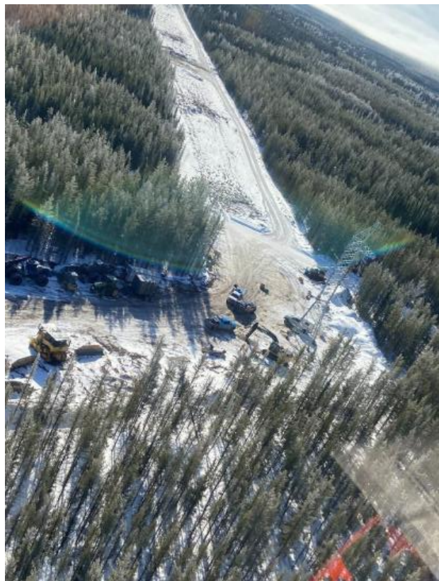
Cleared vegetation along the 40m Right of Way (ROW).
