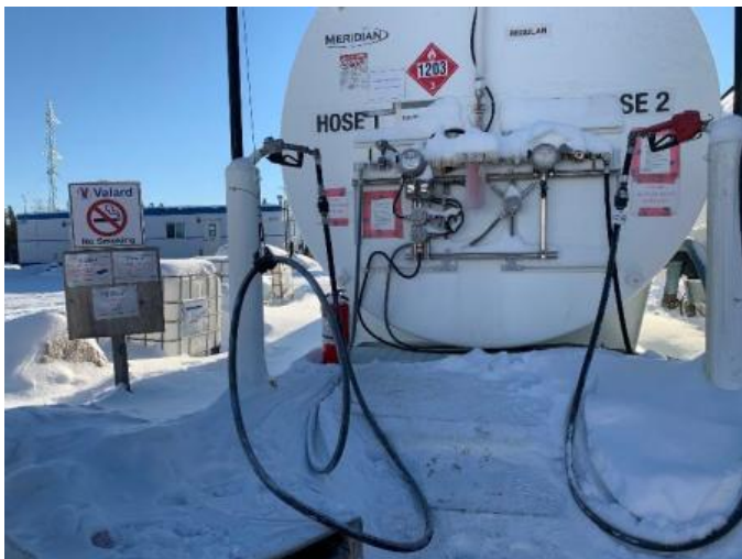
Fuel signage installed at Pipestone Camp fueling area.
