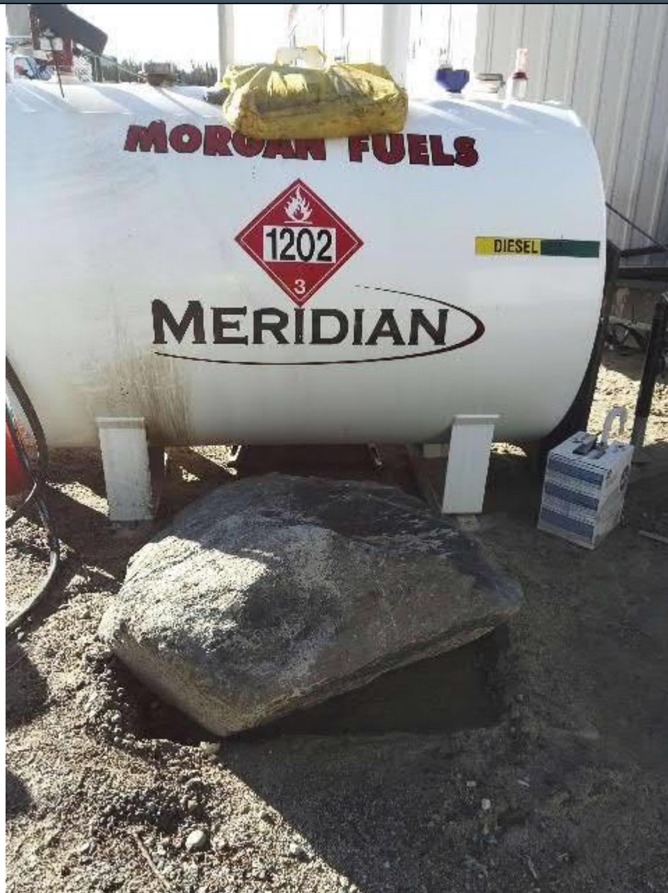
Figure 1: Spill kit at fuel tank
