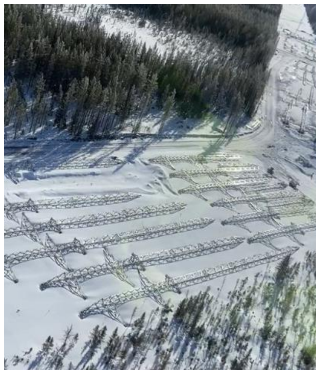
Cleared RoW used as a structure assembly and laydown yard.
