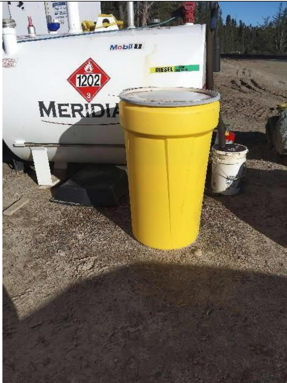
Figure 2: Drip bucket for fuel nozzle is full of water and fuel
