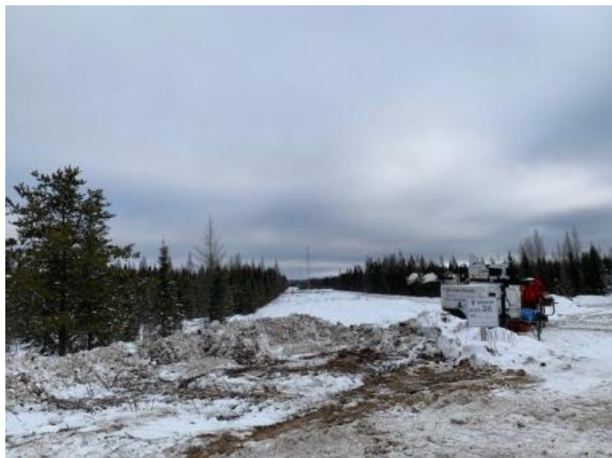
ROW signage present at P1P2 Access 36
