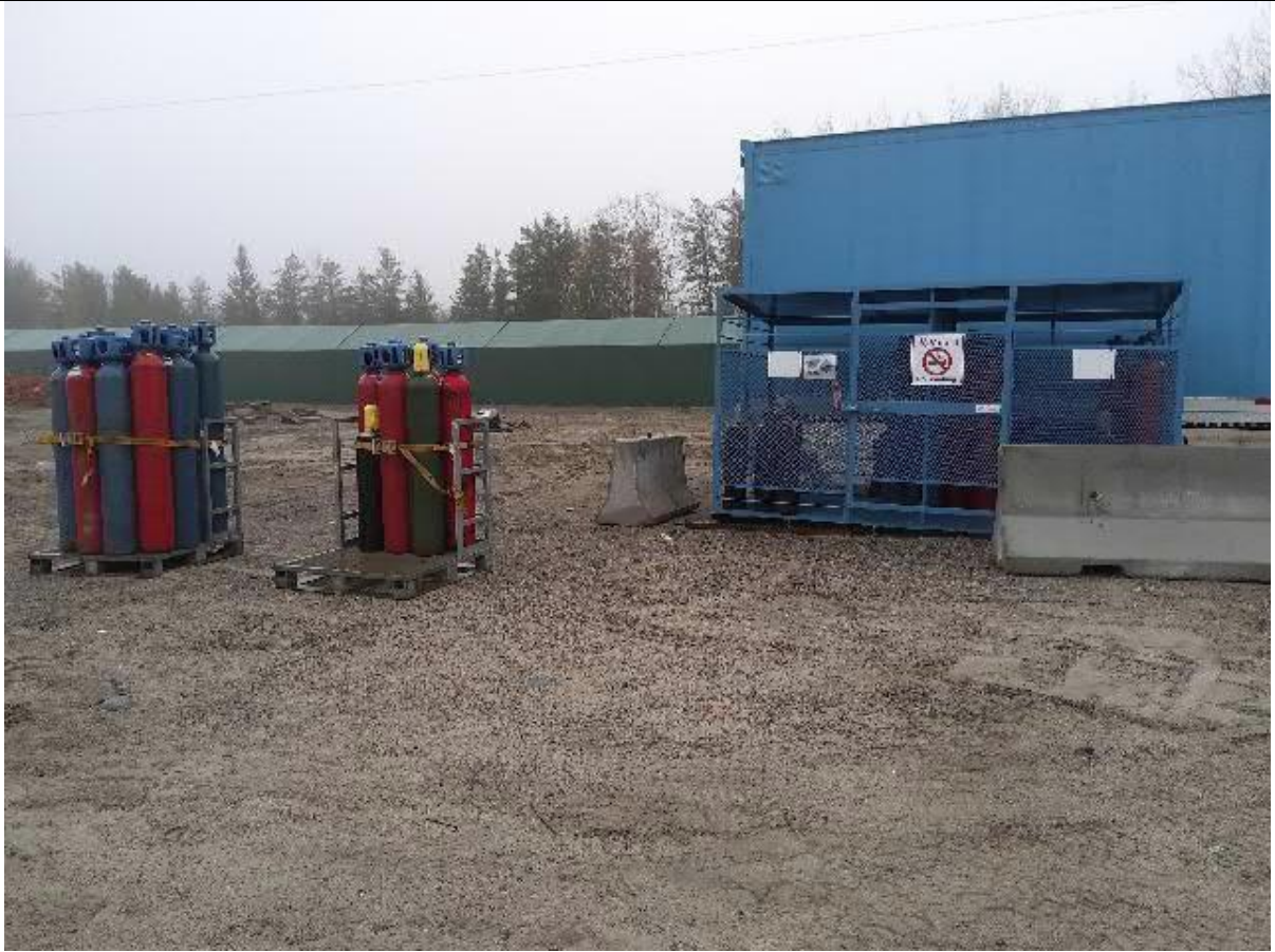
Figure 6: Compressed gas storage
