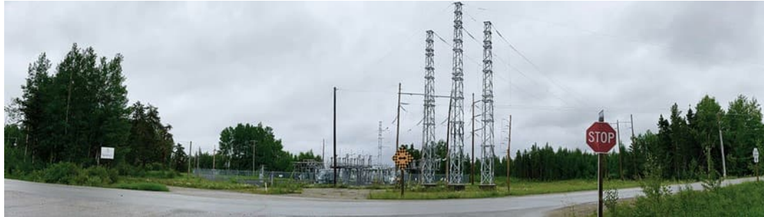
Figure 26: VP9 Site Visit Photo
