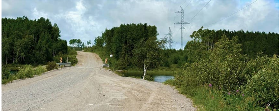
Figure 18: VP6 Site Visit Photo
